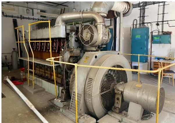
Obr. 35: Dieselagregát
